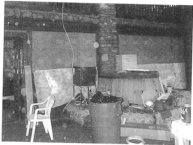
Figure 2. Interior of Gillette Castle during restoration.
